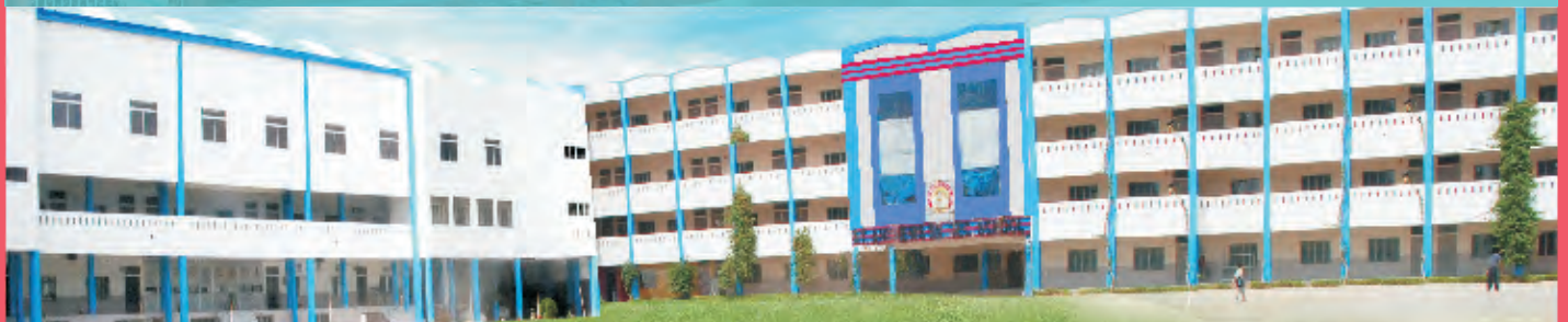
St. Andrews Public School, Kamla Nagar, Agra M.: 9720005927
